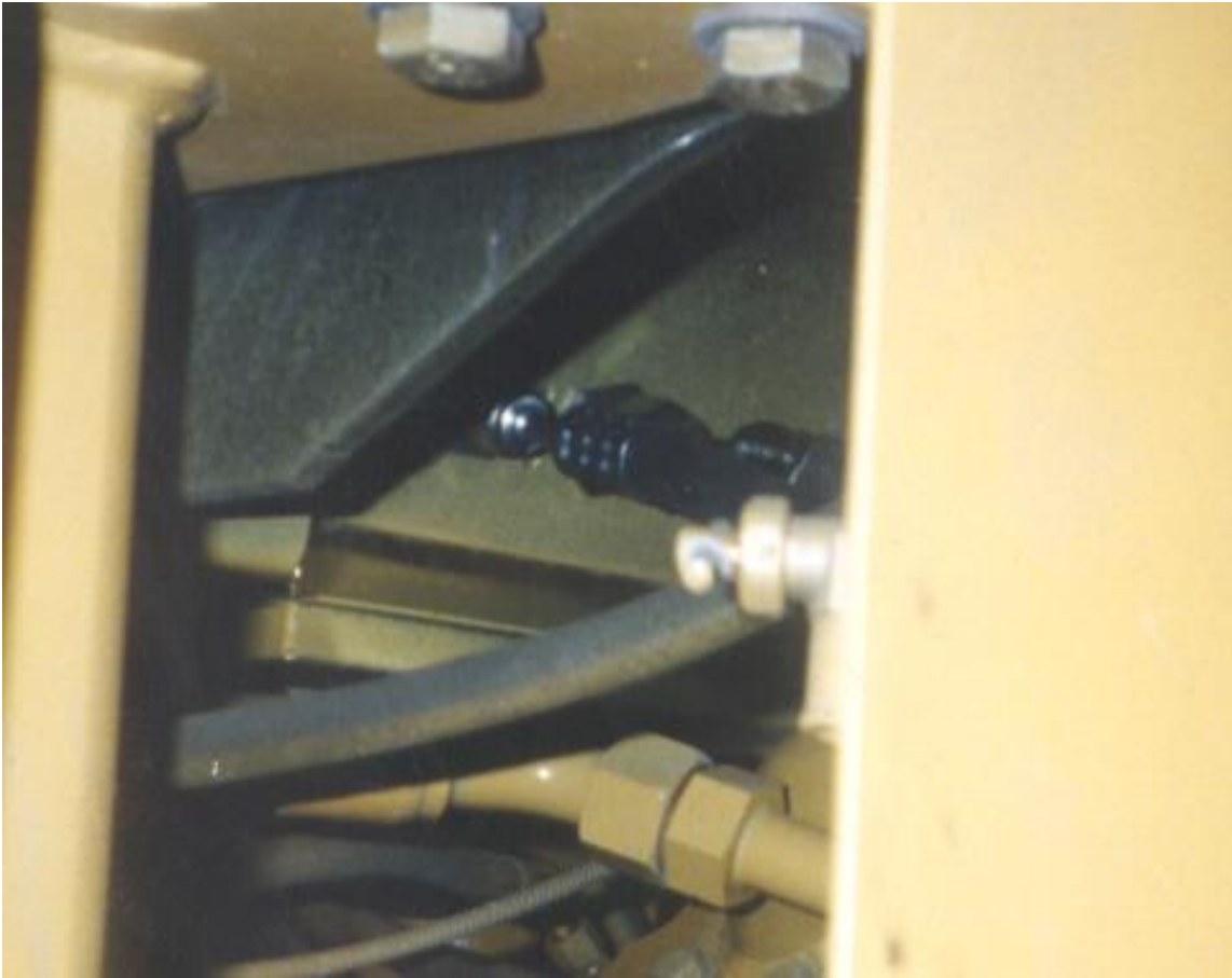
Hose going to back of the cab. Bulkhead fittings are no longer used.
